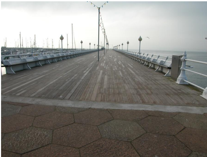
1 Timber boardwalk at Princess Theatre promenade
